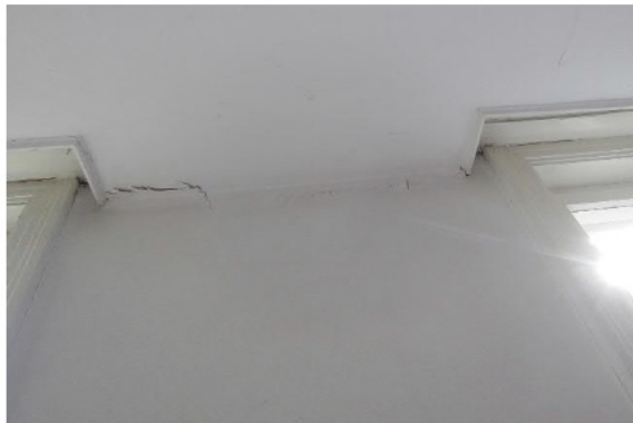
Abb. 109 Riss in Decke
