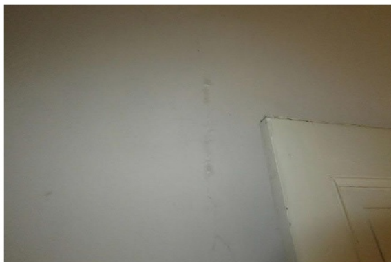
Abb. 116 Trennriss Schornstein
