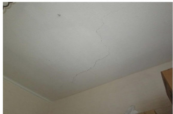
Abb. 125 Riss in Putzdecke
