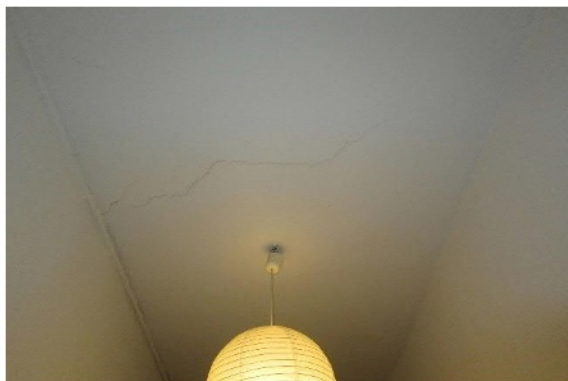
Abb. 128 Riss in Decke
