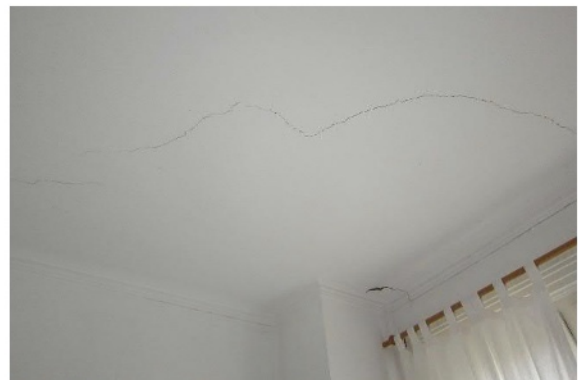
Abb. 137 Riss in Decke
