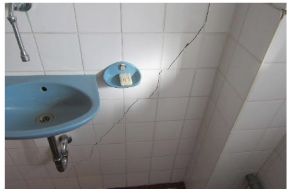
Abb. 63 Riss in Querwand
