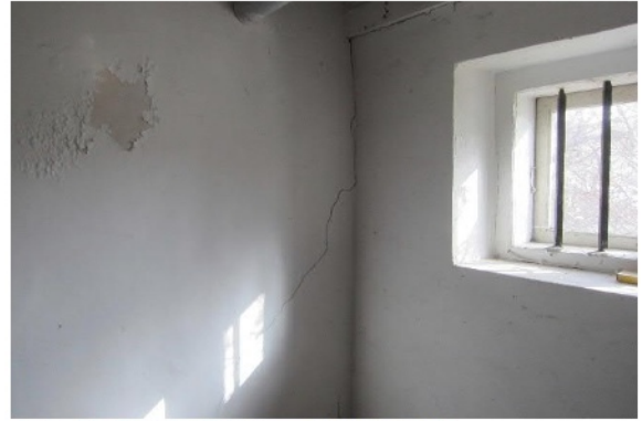
Abb. 57 Riss in Querwand K06 zuK04
